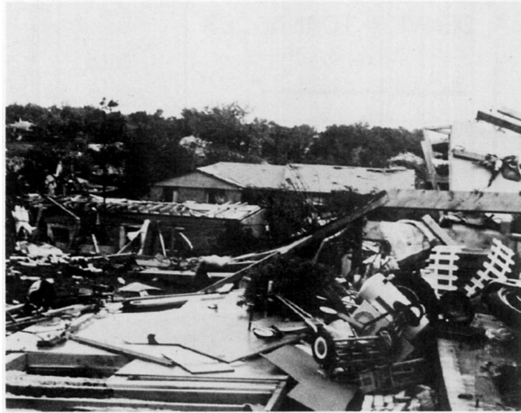
FIG. 2. Photograph of F2 damage from the Thornton tornado.
