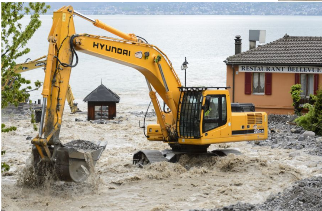
Flooding in St. Gingolphe, Valais May 1, 2015
